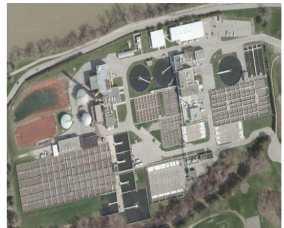
London's Greenway Wastewater Treatment Plant
